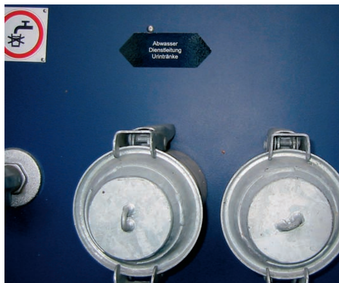
Urine on tap: At the withdrawal point, urine collected in Forum Chriesbach can be pumped into a tanker as required (Photo Karin Güdel)
