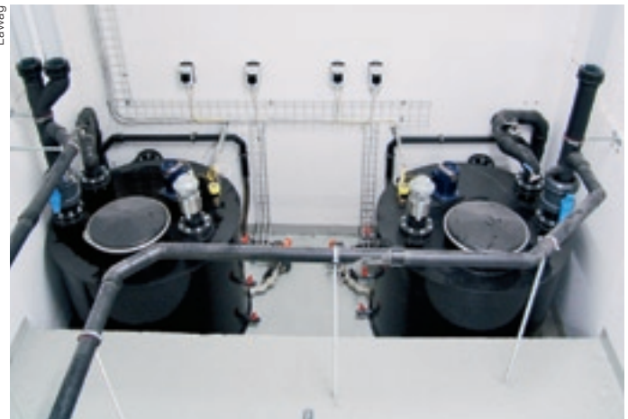
At Forum Chriesbach, urine is also separately collected from male and female users. The new Eawag headquarter building is fitted with NoMix toilets throughout.
